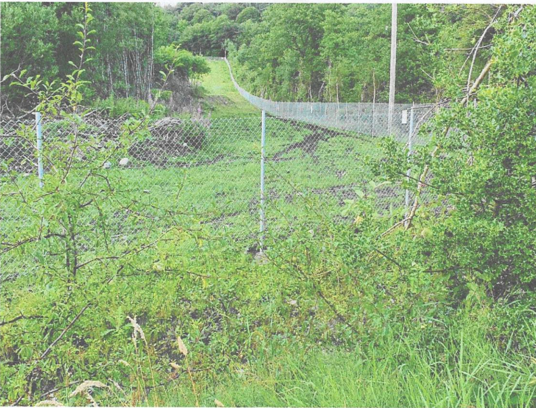
Image 6.16 New fence erected around perimeter of quarry
