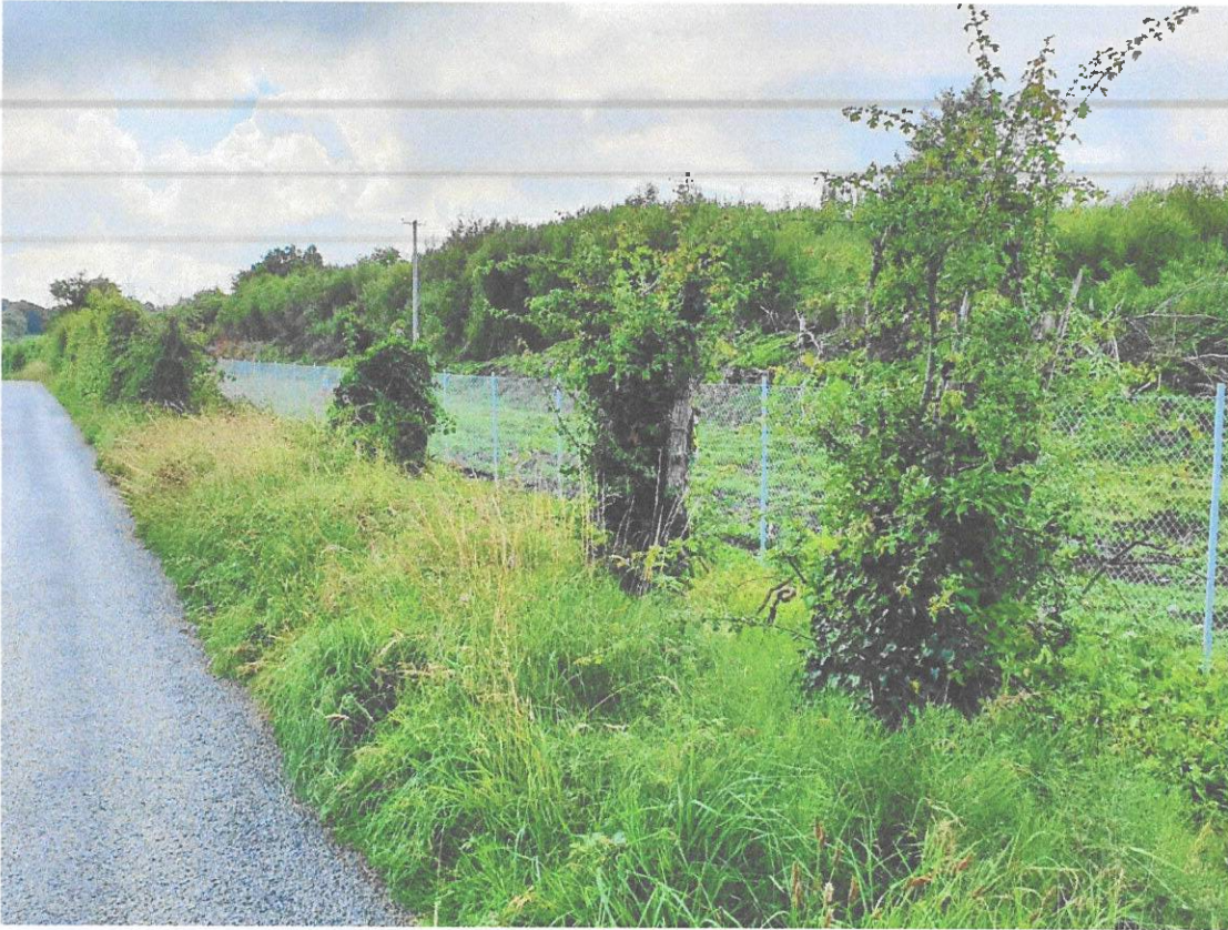
Image 6.15 New fence erected around perimeter of quarry
